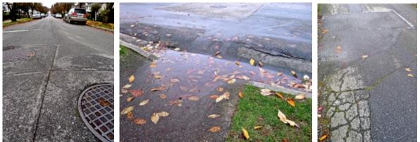
The state of the asphalt along a stretch of the site of act 2, "The Swamp." Notice the buckles, bends, and cracks in the pavement as of November 2012. Photographs by author.
